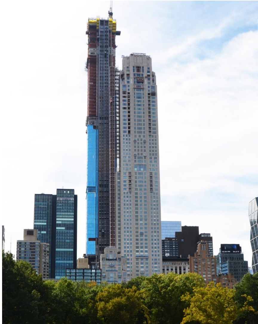
220 Central Park South
