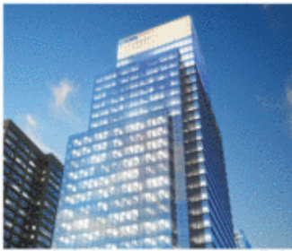
CEB Tower at Central Place
