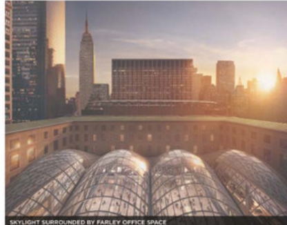
SKYLIGHT SURROUNDED BY FARLEY OFFICE SPACE
