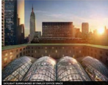
SKYLIGHT SURROUNDED BY FARLEY OFFICE SPACE
