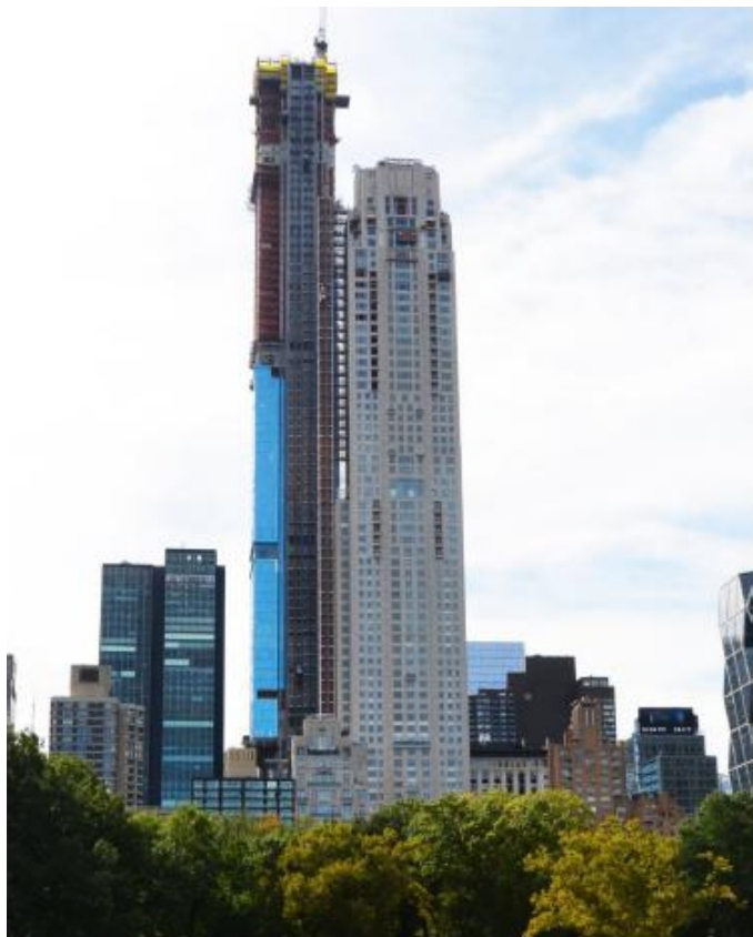
220 Central Park South
